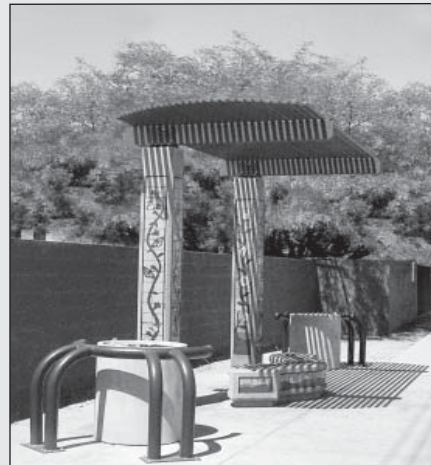
New bus shelter at the corner of Broadway and Macdonald in Mesa.
