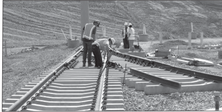
First METRO tracks being laid south of Washington and 48th streets.
