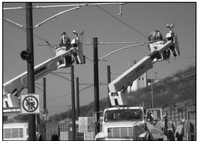
Contractor Mass Electric installing wire
