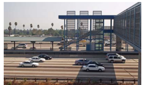
Sierra Madre LRT Station - Gold Line, Los Angeles, CA
